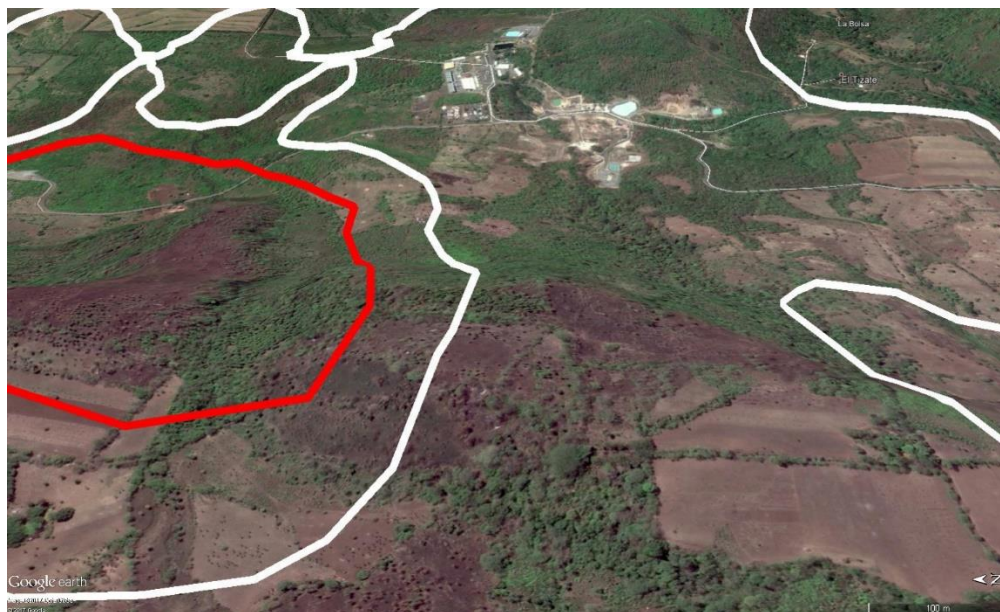
Figure 13. View of the El Tizate production area, looking eastwards and down slope into the El Tizate production area valley from the rim of the Los Tablonos fault. Recharge flows down toward El Tizate from Los Tablonos and the higher elevation catchment to the west. Recharge forms a reservoir at the El Tizate topographic low; note the hill immediately to the east of the production area prevents recharge escaping further east. Recharge is heated and acidified (by CO 2 , H 2 S), and alters volcanics to clay. White boundary is the LFZ that results from the clay cap. Red boundary encloses HFZ to the north, located on adjacent catchment. Image with vertical exaggeration from Google Earth.
